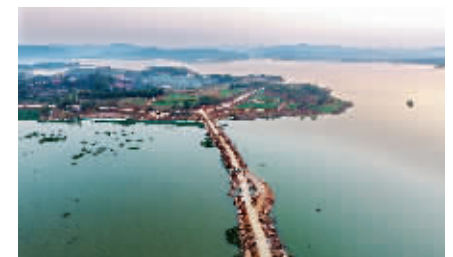
Path linking to Luoyan Island
