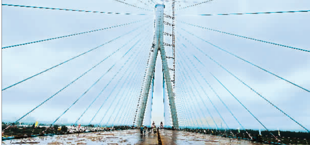
Zhuankou Yangtze River bridge under construction Photo by Hu Jiusi
